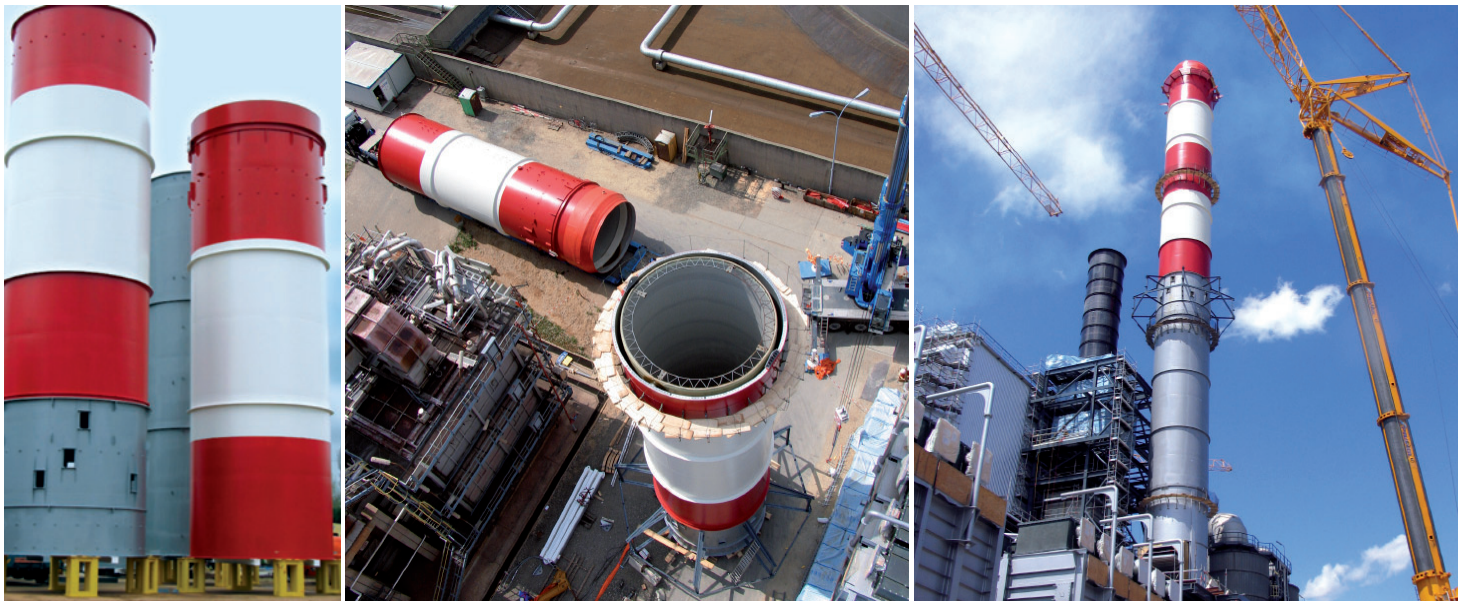
From left to right: Installation steps through to the finished chimney.
